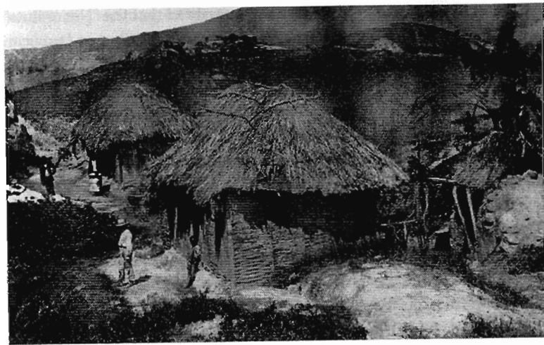
Figure 2 Wattle-and-daub houses with thatched roofs, probably very similar to ones found during the slavery period. Judging by the topography, the photo was taken in the Scotland District, quite possibly Chalky Mount in St Andrew (as suggested by the packed "beehive" potter's kiln in the lower right hand corner). The photo was taken by the well-known American photographer Frank Carpenter, probably in the late nineteenth or early twentieth century (he died in 1924), judging by his various publications on his early travels to the West Indies and South America. [Courtesy, Library of Congress, Prints and Photographs Division, Frank and Frances Carpenter Collection, LC-USZ62-95078.]
