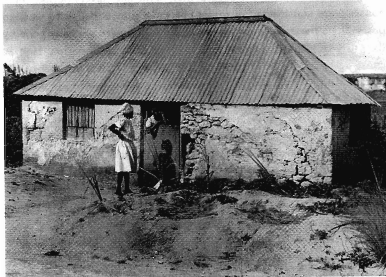
Figure 5 House of rubble stone construction, with limestone exterior plaster and galvanized iron hip roof. In earlier days, the roof would have been thatched. The photograph is undated, but was perhaps taken in the 1940s or 1950s. The location is unknown. The photo was given to Handler by Maggie Goodridge in December 1983.
