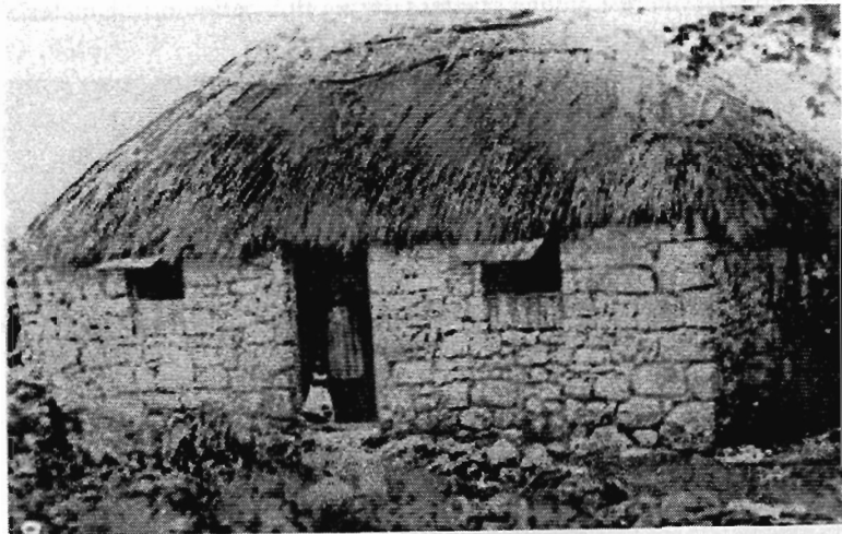
Figure 3 Stone house with thatched roof. The poles on top held down the roof thatch. Although this photo was probably taken in the late nineteenth or early twentieth century, the house shown appears to be very similar to the type of stone house found in the later years of the slavery period. [Courtesy, Barbados Department of Archives, Laborde Collection, # 8.]
