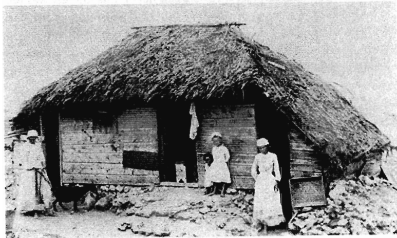
Figure 4 Wood plank house with thatched roof, June 1907. This house probably closely resembles the wood plank house found during the later years of the slavery period. [Courtesy, Barbados Department of Archives, Registered photos, 1905-1907, #81.]
